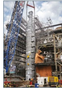
Positioning and installation of de-ethanizer column with 650 Ton Crawler Crane
