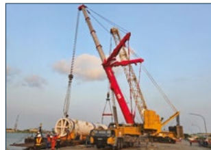
Off-Loading LHU Column from a vessel
