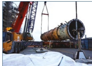
Decommissioned column being transported on an SPMT
